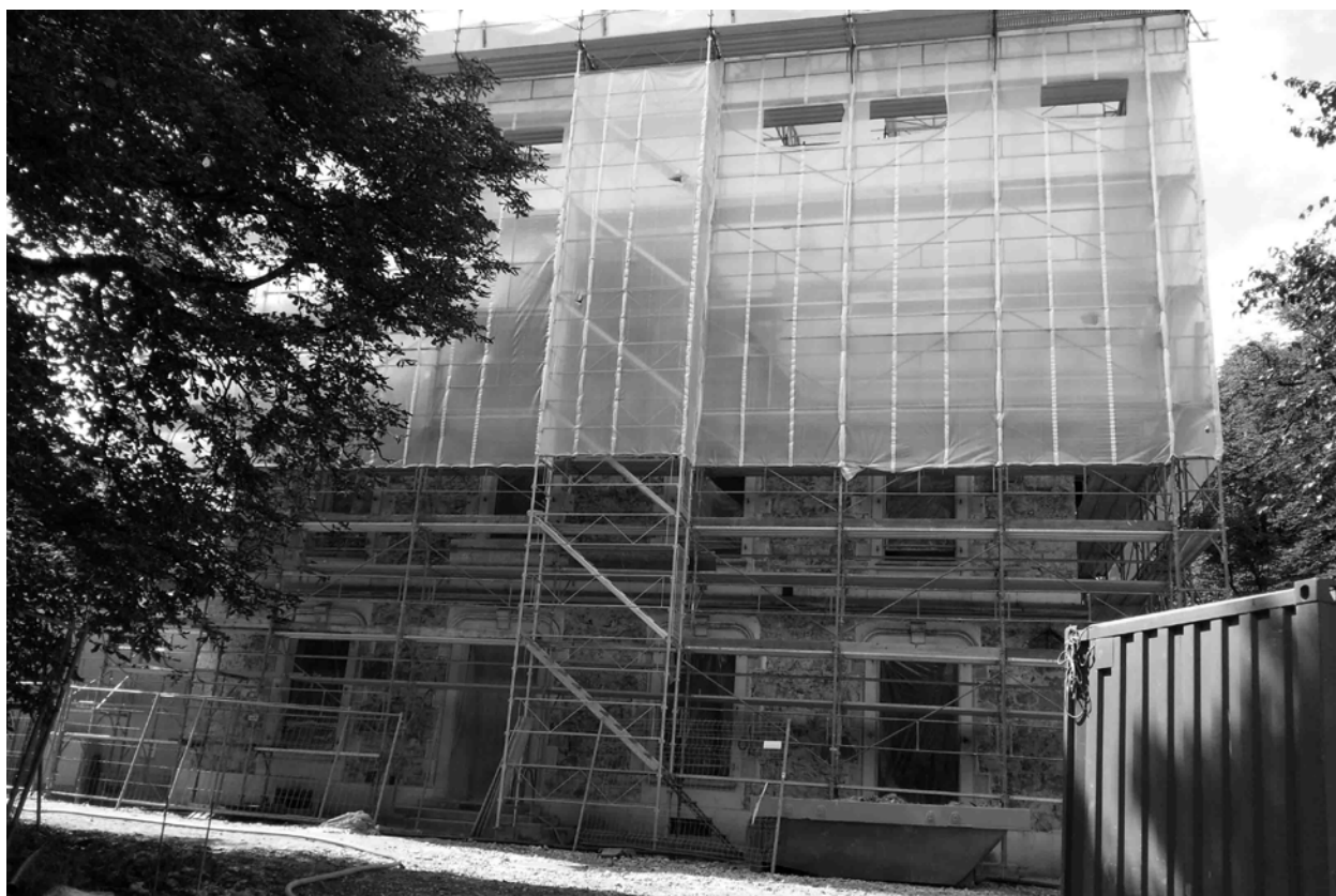
Renovation of Geneva Call's new office in Chêne-Bougeries © Geneva Call
